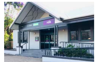
8 Centrelink and Medicare Offices
