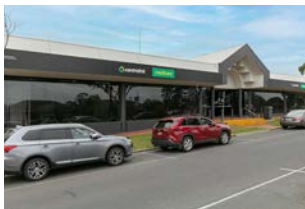
13 Centrelink and Medicare Offices
