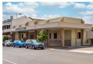
2 Centrelink and Medicare Offices
