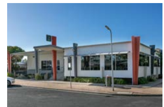
12 Centrelink and Medicare Offices
