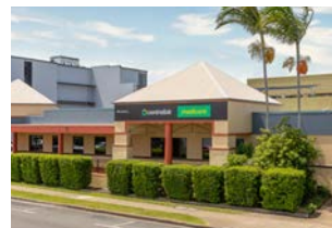
3 Centrelink and Medicare Offices
