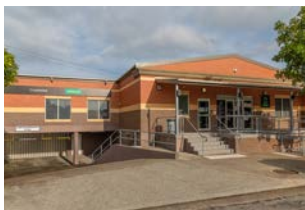
9 Centrelink and Medicare Offices
