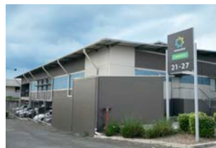
6 Centrelink and Medicare Offices
