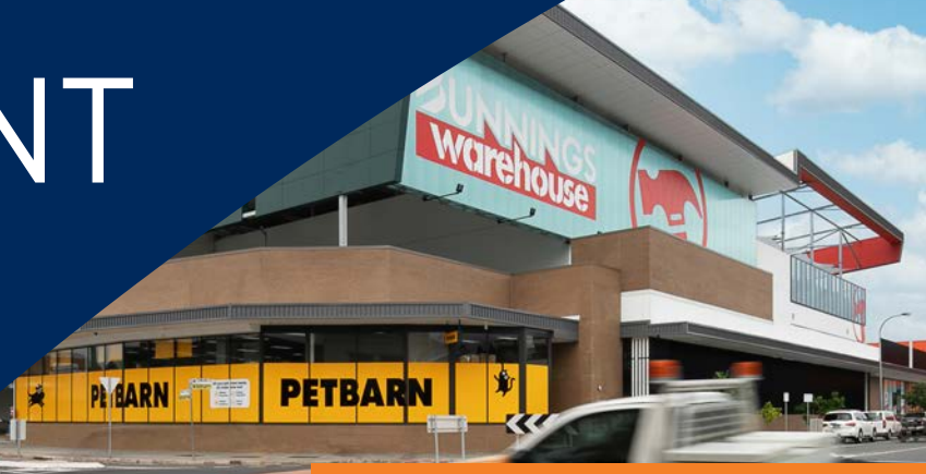
Bunnings Warehouse and Petbarn at Newstead, QLD.
