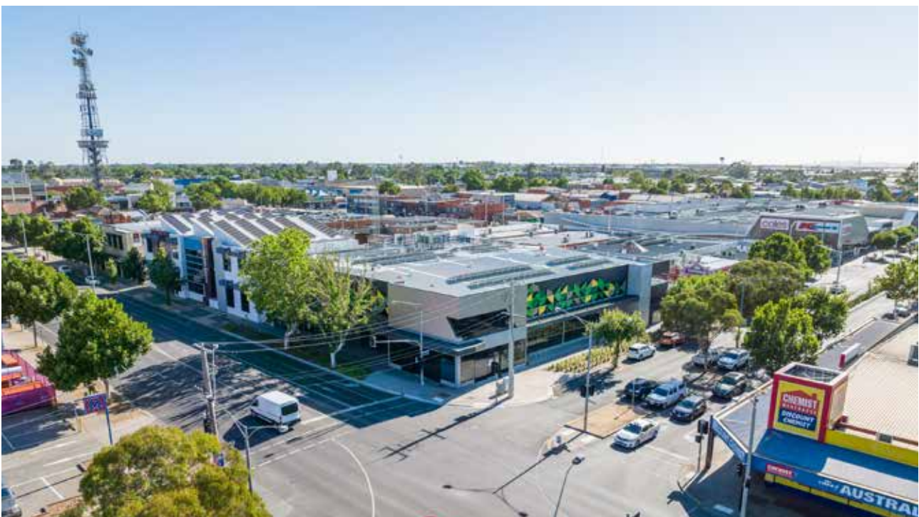
Dept. of Justice and Court Services, Shepparton VIC - A property held in the MPG Essential Services Property Trust
