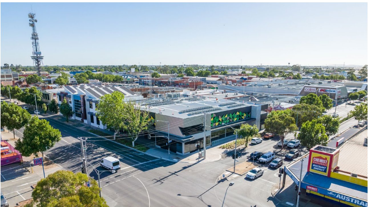
Dept. of Justice and Court Services, Shepparton VIC - A property held in the MPG Essential Services Property Trust
