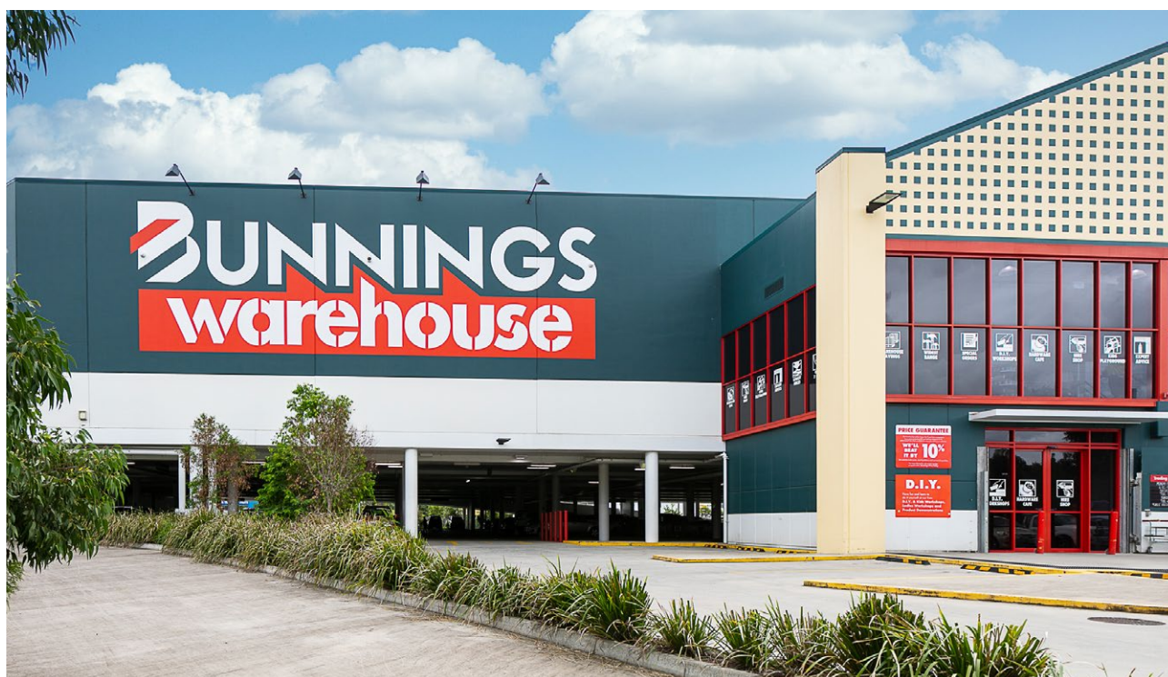
Bunnings Warehouse, Bundamba, QLD
